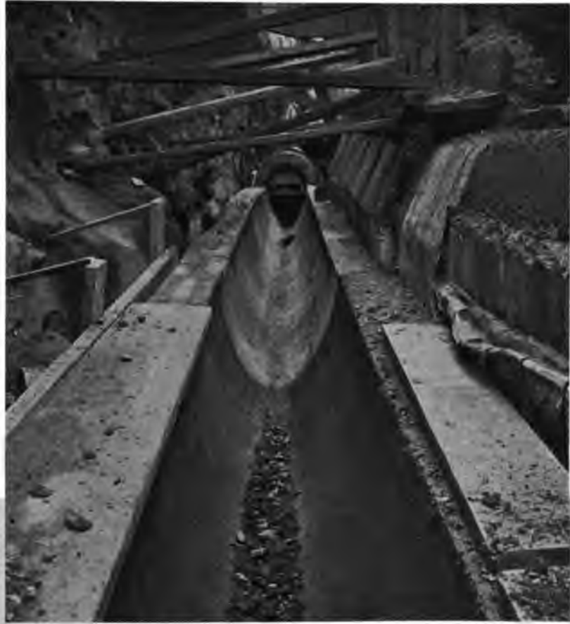
CONCRETE SEWER BACK OF SIDE WALL, BROADWAY AND 56TH STREET
